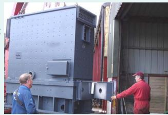
Since then work by Contract Services has continued apace to install the boiler and connect the pipes which will carry the heated water around the greenhouses in preparation for a 'topping out' ceremony in July.
