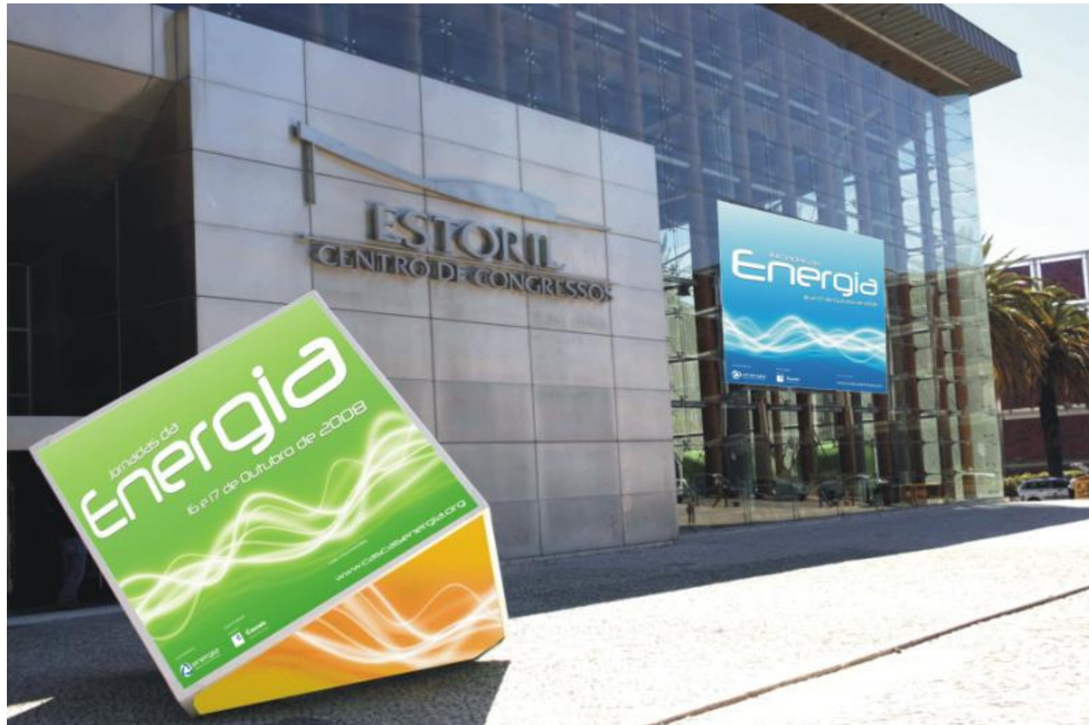
Exterior decoration of the Estoril Congress Center
